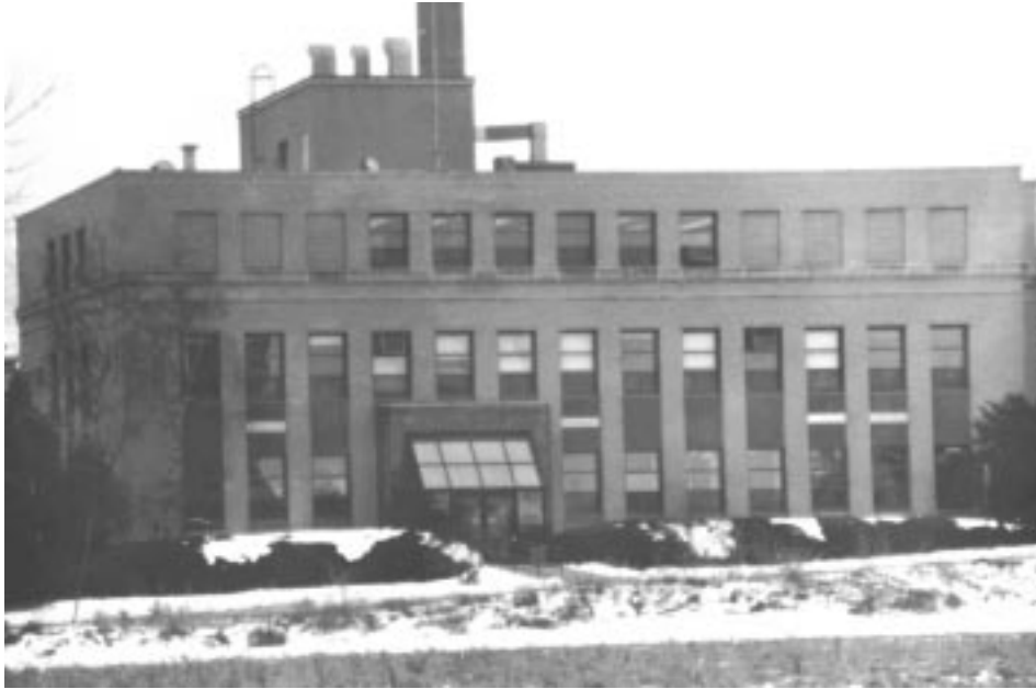
Fig. 1. 1995. The old WARF building, built in 1947 it is three stories of concrete and steel over a full basement. It is skinned with face brick and granite trim. [Author Photo, AP-26]
